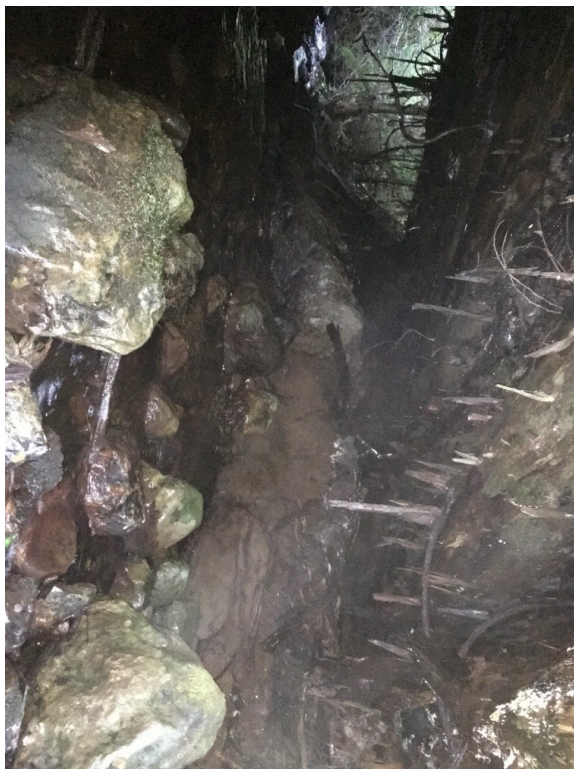
Right Bank Abutment when facing downstream
