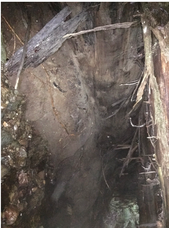
Left Bank Abutment when facing downstream
